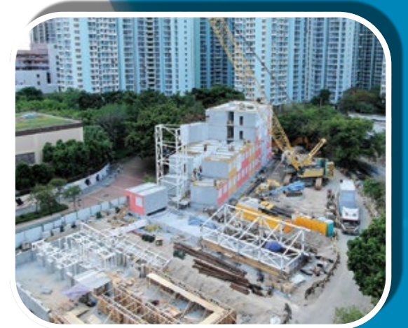
MiC Modules Installation on Site
