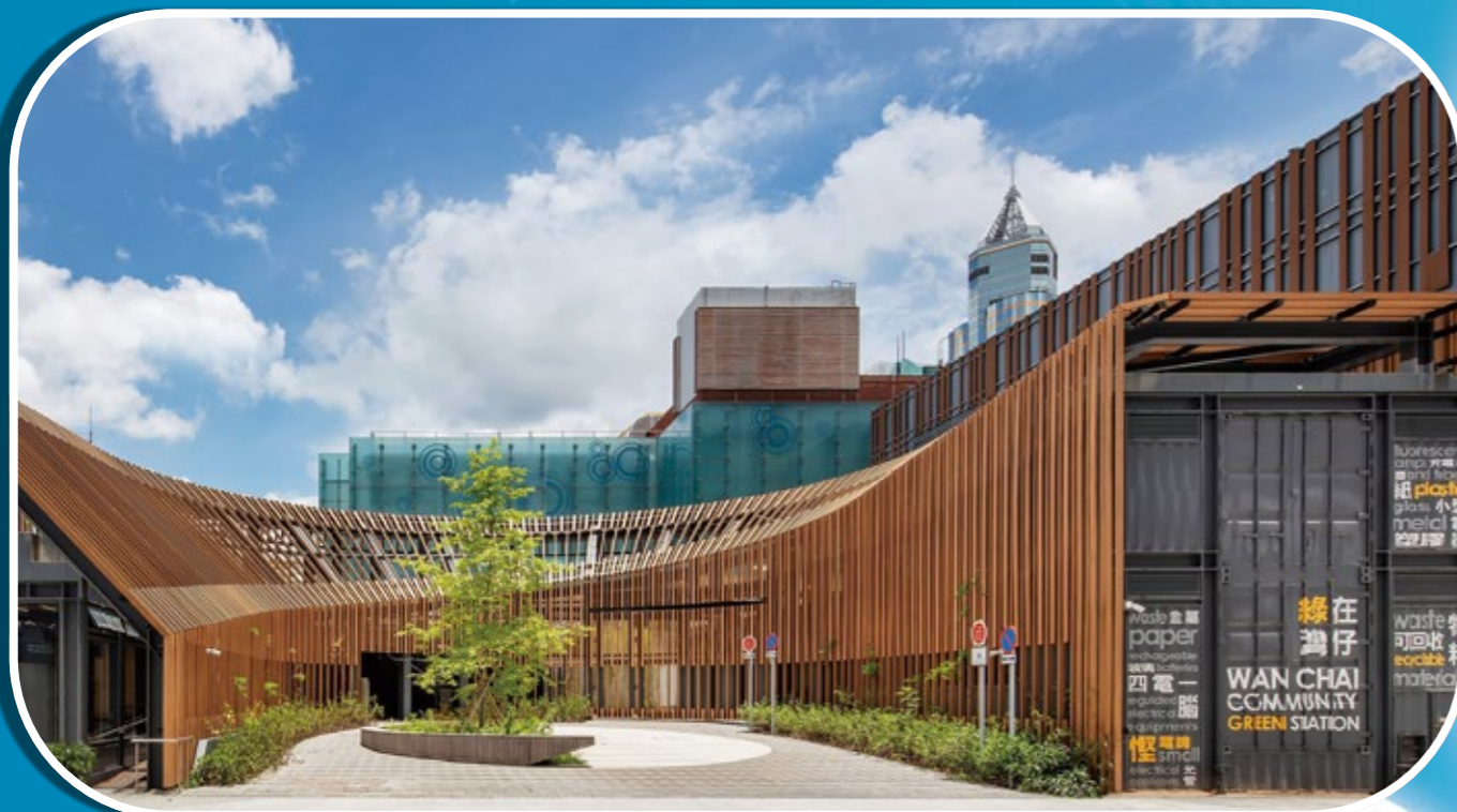
Unique architectural design of Green@Wan Chai serving as iconic building and educational centre.
