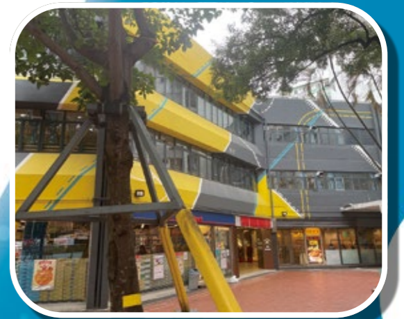
Kai Yip Shopping Centre - Facade and Addition of Windows
