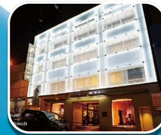
The old facade design resulted in light pollution issues in the neighbourhood.
