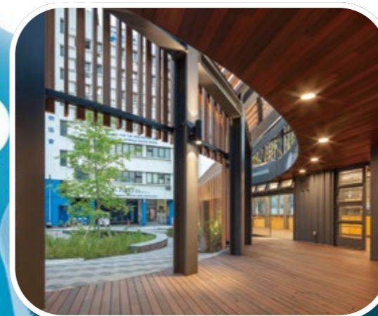
Green design including Glass Reinforced Plastic (GRP) trellis roof as thermal buffer, rain garden, energy efficiency provisions, etc..
