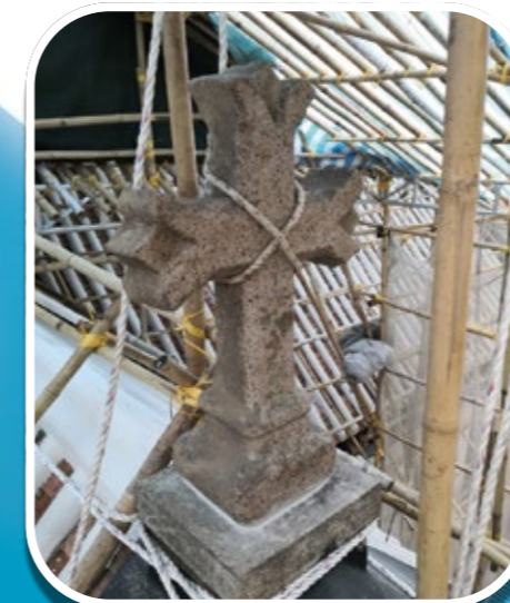
Restoration of Historic Feature
