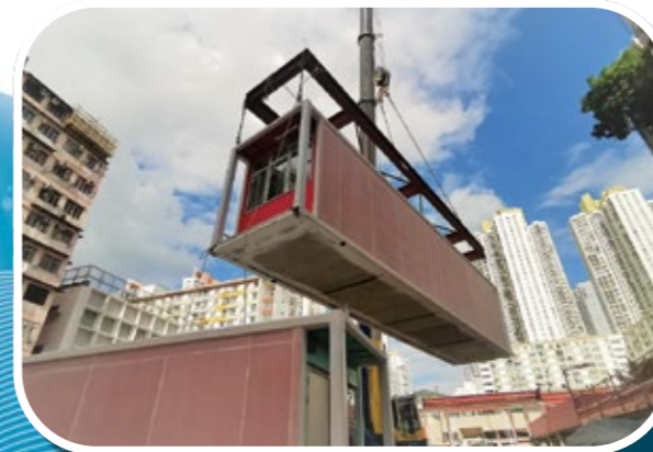
Hoisting of MiC Module.
