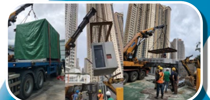
Delivery of MiC Modules on Site
