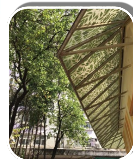
Refurbished polycarbonate canopy to blend into the surrounding environment
