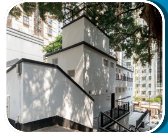
The public toilet and bathroom seamlessly integrates with its surrounding neighbourhood, enriching its overall character
