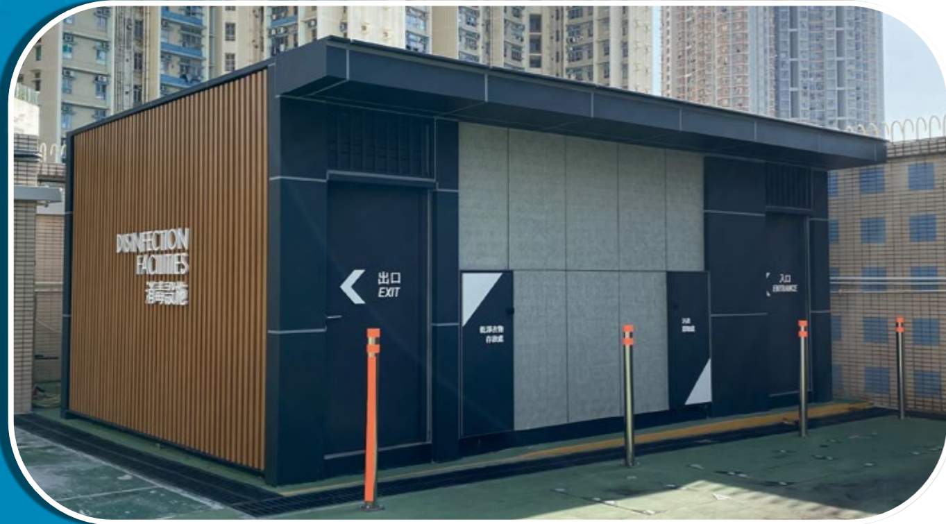
Overview of Disinfection Facilities in Lam Tin Ambulance Depot
