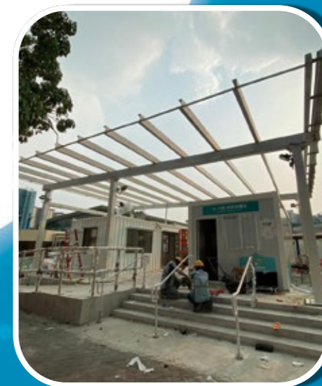
Installation of handrail in progress
