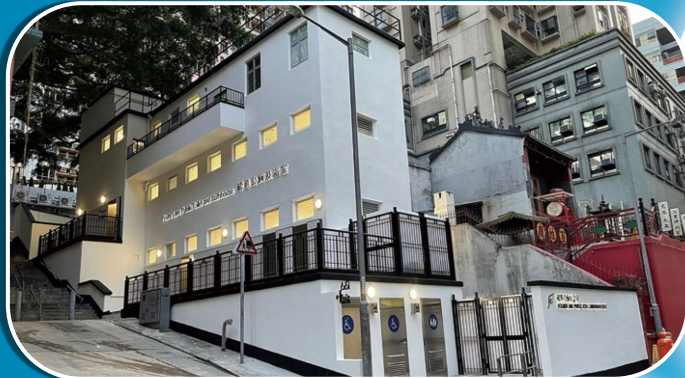
Overall external view of Pound Lane Public Toilet and Bathroom
