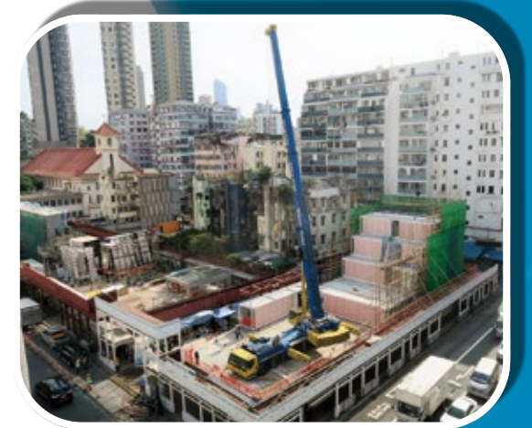
MiC Module Installation on Site
