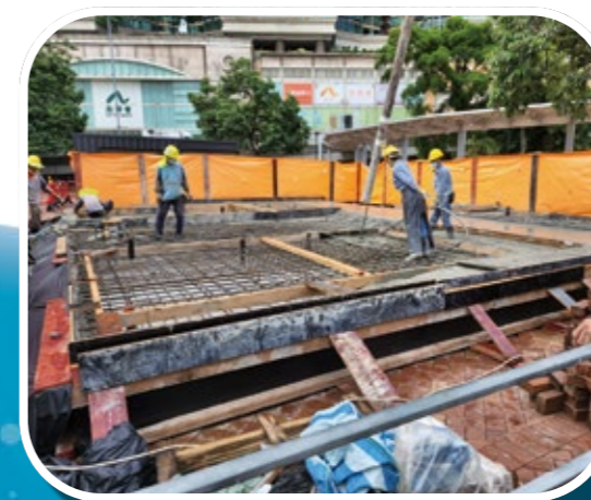
Concreting work of foundation
