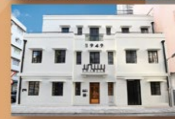
Tai Hang Fire Dragon Heritage Centre, Hong Kong Ceramic Breathable Coating System
