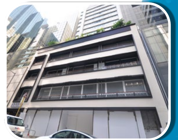
The architectural features were inspired by the "Tong Lau 唐樓" style - canopy, balustrade & column
